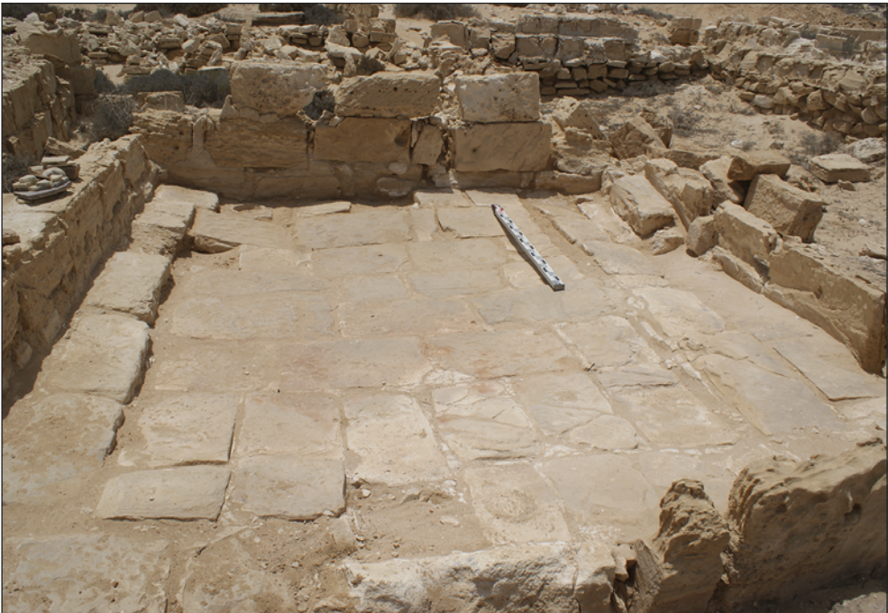
Fig. 7. Building H41, unit 5, view from the north
