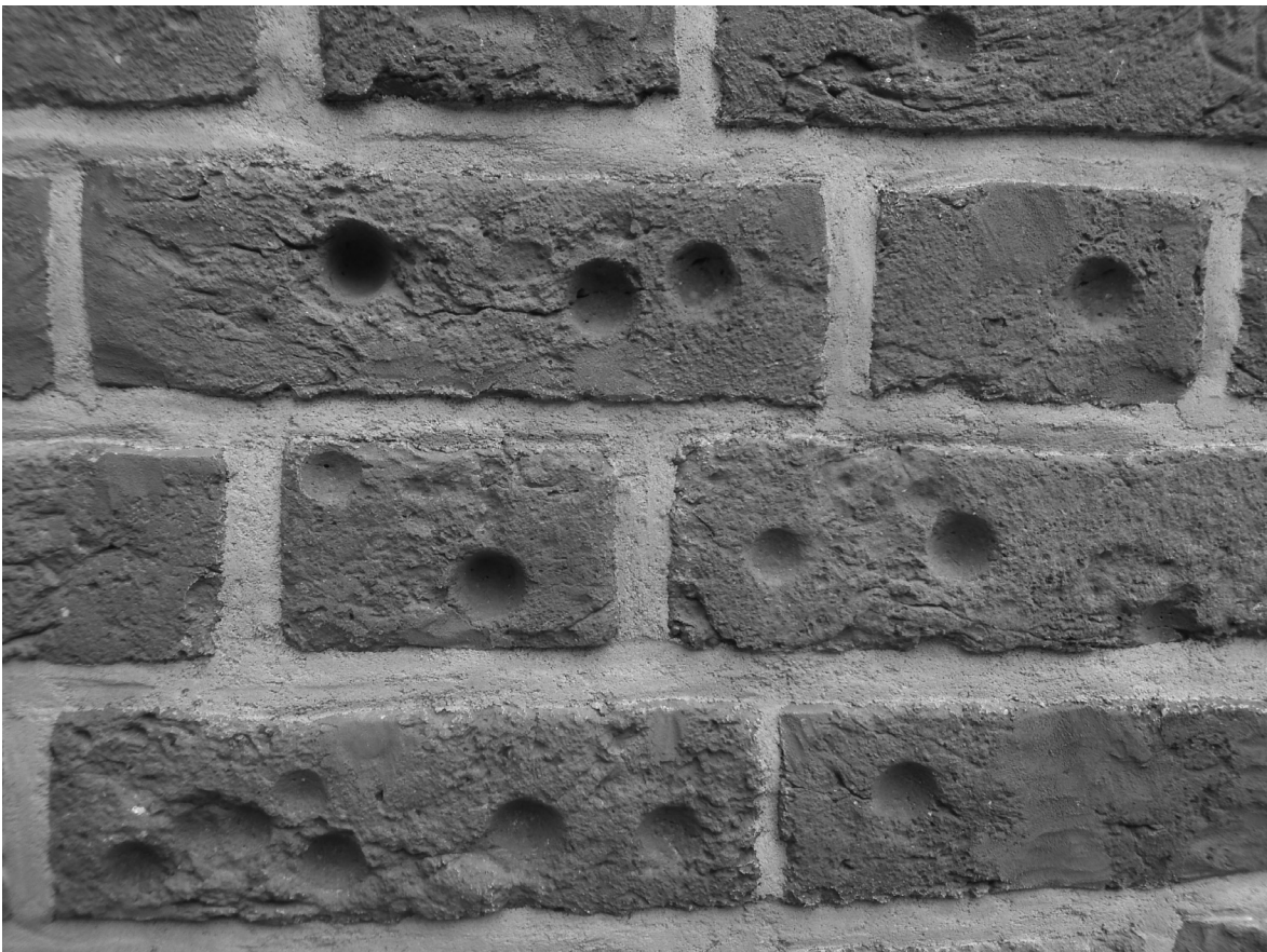
Fig. 44. Penance holes and shape of willow leaves signs (source: Ł. Karol's archive)
