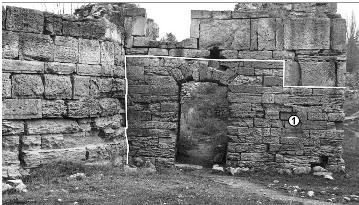
Fig. 2. Curtain 19, interface with the earlier Turret XVI. View from the outer ward (R. Karasiewicz-Szczypiorski). 1 – surviving part of the defensive wall from the earliest building phase (Hellenistic wall).
